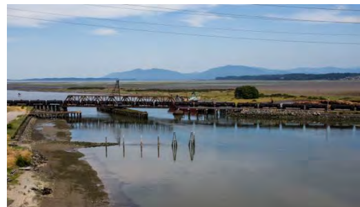
The Anacortes Subdivision contains a trestle and a swing bridge—the Swinomish Channel Swing Bridge.
