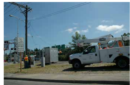
Public works crew checking signal phasing
