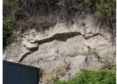
Landslide area within the project vicinity
