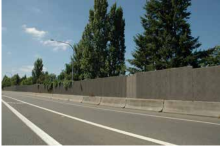
Existing noise wall on I-405 near NE 30th
