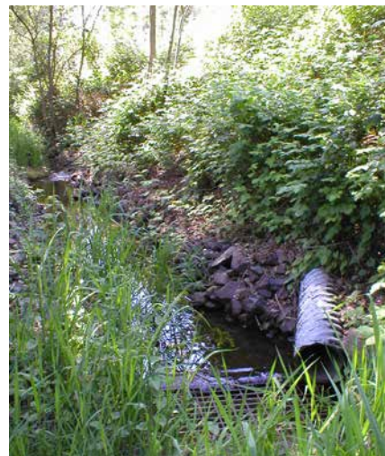
Stream culvert in the study area
