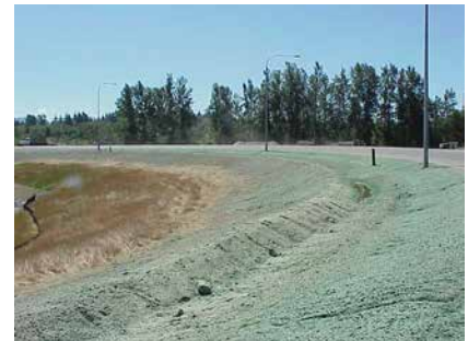
Ecology embankment under construction
