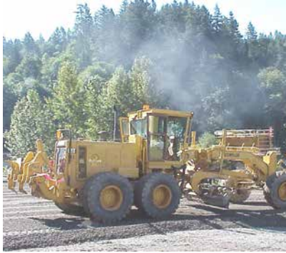
Grading to finish roadway subgrade
