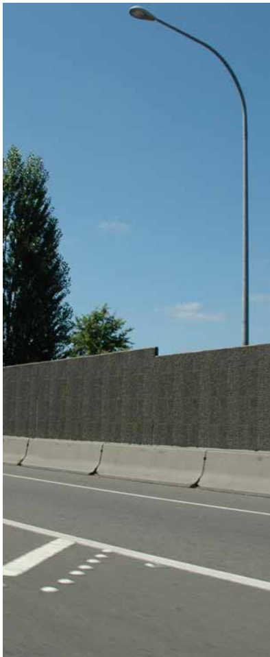
Existing noise wall
