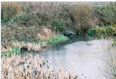
Culvert in the project area
